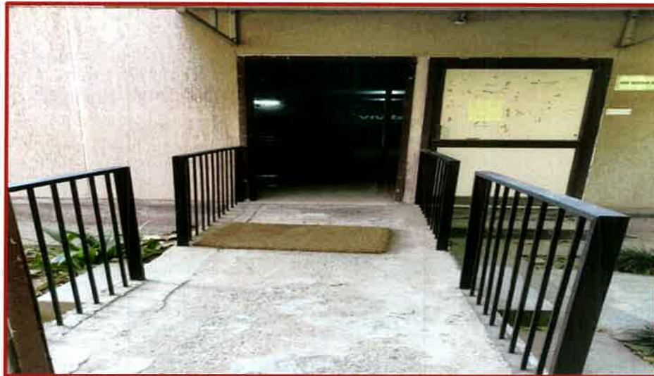
Fig. 1b. Ramp at the entry of New Seminar Room
