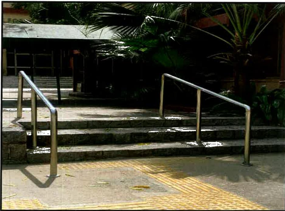
Fig 2b. Railings at the entry to the plaza
