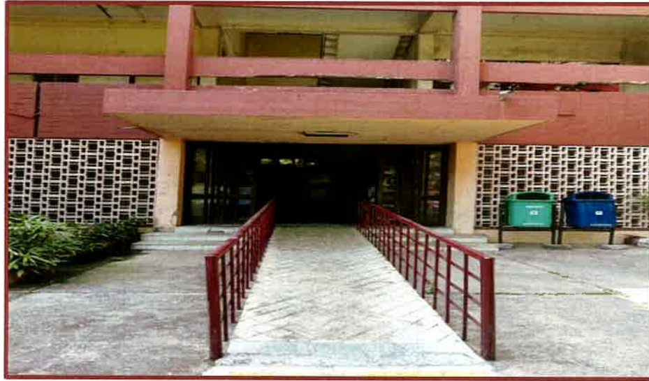
Fig. 1a Ramp at the entrance door
